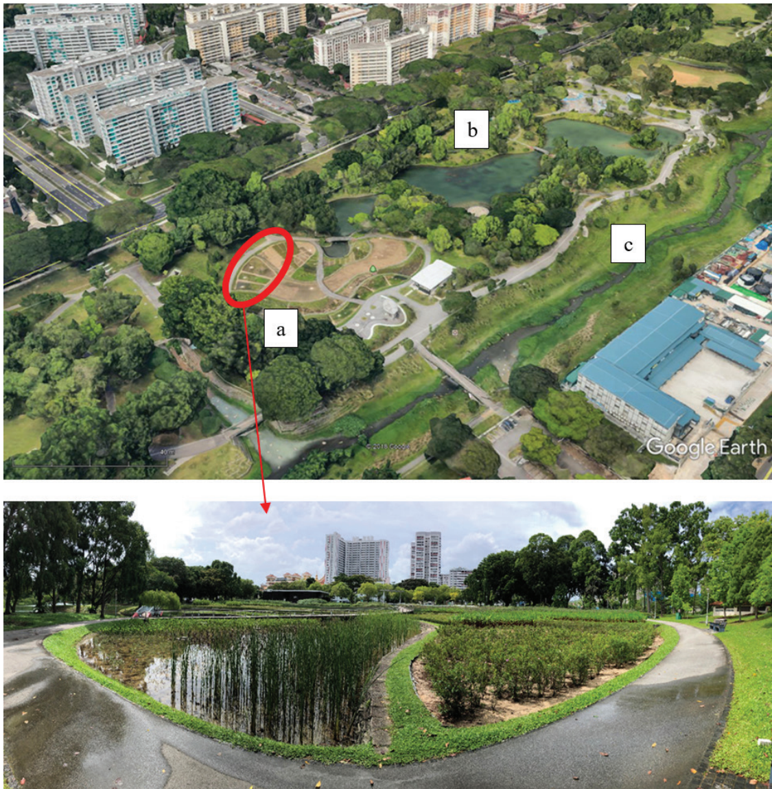
Figure 4: Cleansing biotope (above) in upper Bishan Park (a), with recirculating ponds (b) and Kallang River (c). This location is upstream of the area shown in Figure 3. Google Earth Pro, imagery date 1 February 2019, Bishan Park, Singapore, accessed 9 September 2019. Photo of the cleansing biotope (below, photo by the authors).
