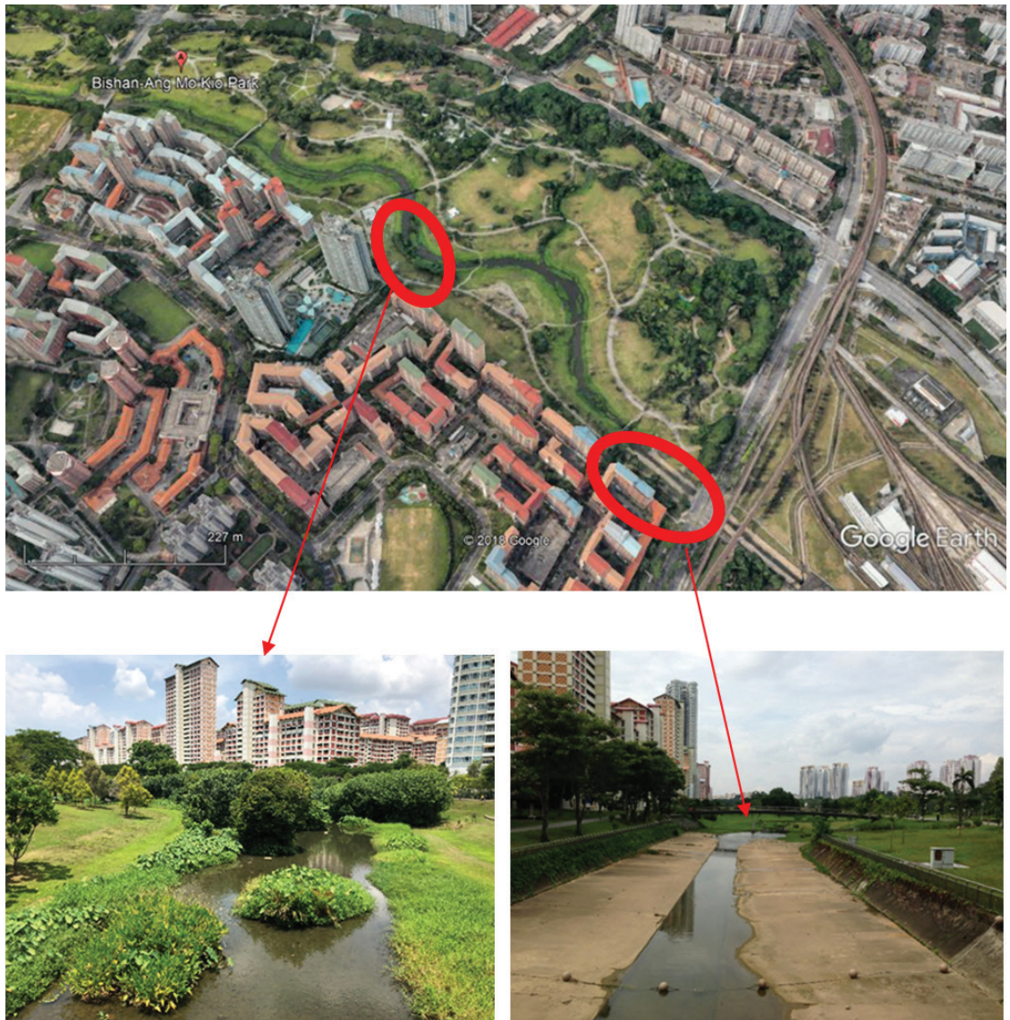
Figure 3: Bishan Park naturalized channel and floodplain (top, Google Earth Pro, imagery date 1 February 2019, Bishan Park, Singapore, 9 September 2019) and corresponding in situ photos of concrete channel draining the naturalized section of the park (lower right). The upstream park channel was concrete like this prior to 2012. Re-constructed (naturalized) river with mid-channel bars and functioning floodplain (lower left) (lower photos by the authors). HDB flats overlooking Bishan Park are observed in the background.
