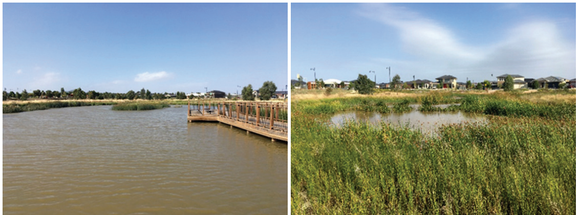
Figure 2: Grand Lakes constructed wetland with boardwalk (left) and sedimentation cell (right). Photos by authors.
